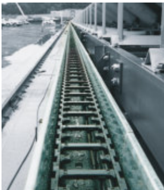
Conveyor belt in quarry. Application with travel distance of 179 m, travel speed 67 m/min., fill weight 8 kg/m
