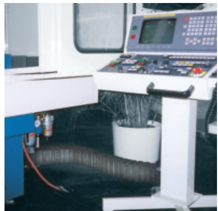
Triflex® 332 as unsupported link from machines to control desk
