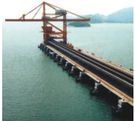
Many successful RoI E-Chain® applications, i.e. one of the igus® longest travels at the moment on 2 ship unloaders in Malaysia, both equipped with a RoI E-Chain® at 441,3 m travel length
