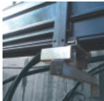
Example of mounting the console on jibs
